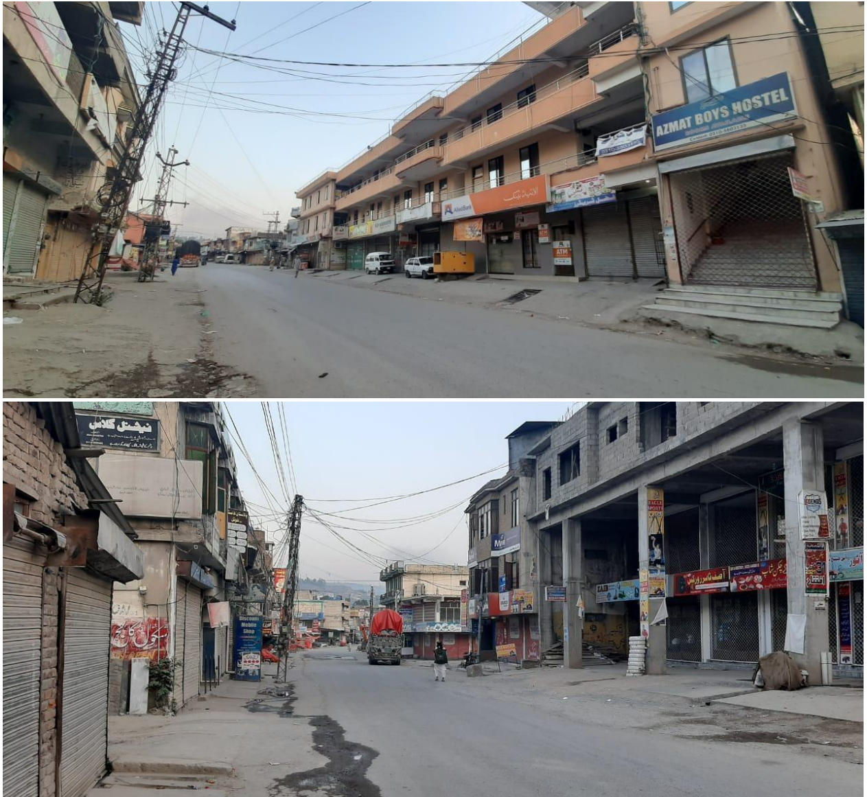
Figure # 7 & 8: Building façade and visual height
